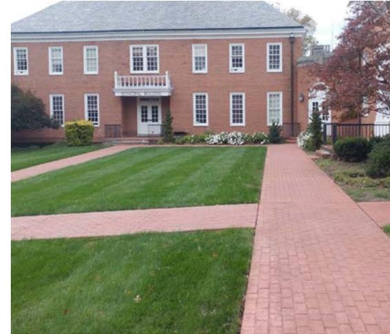
Five rain gardens can be installed in the turfgrass areas around the building to capture, treat, and infiltrate stormwater runoff from the roof of the building. A preliminary soil assessment suggests that more soil testing would be required before determining the soil's suitability for green infrastructure.
