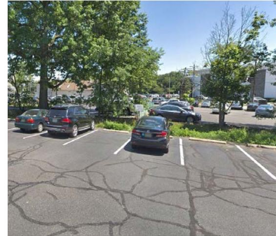
A section of pervious pavement can be installed in the parking lot to capture and infiltrate stormwater runoff from the parking lot. A preliminary soil assessment suggests that more soil testing would be required before determining the soil's suitability for green infrastructure.
