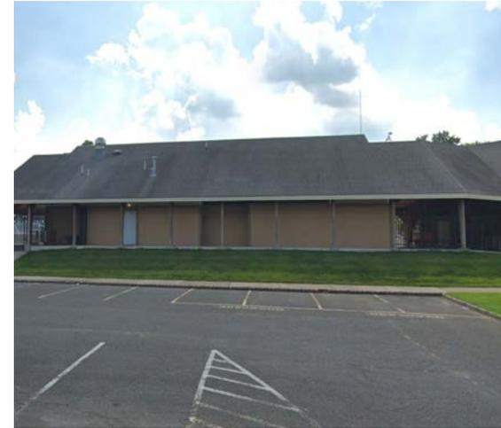
Large rain gardens can be installed in the turfgrass island dividers of the parking lots. A smaller rain garden can be installed adjacent to the building to manage stormwater runoff from the rooftop. Additionally, pervious pavement can be installed in a section of parking spaces to capture the remaining stormwater runoff from the surrounding asphalt. A preliminary soil assessment suggests that more soil testing would be required before determining the soil's suitability for green infrastructure.
